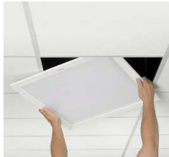
Grid ceiling installation
