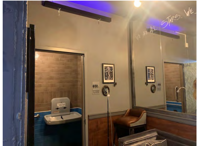
Photo 8: View of the UVC lamps installed along the walls in front of the restroom.
