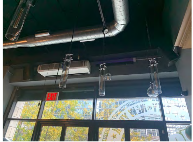
Photo 6: Representative view of the UVC lamps installed along the perimeter walls of the Lounge Area.
